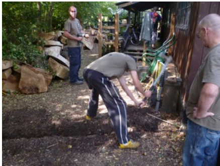
LWT team install electrical cabling for WNT outdoor screens
