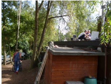
Jamie Griffiths and Rob Scharein install complex 'La Wefan'
