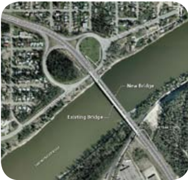
Simon Fraser Bridge, Prince George
